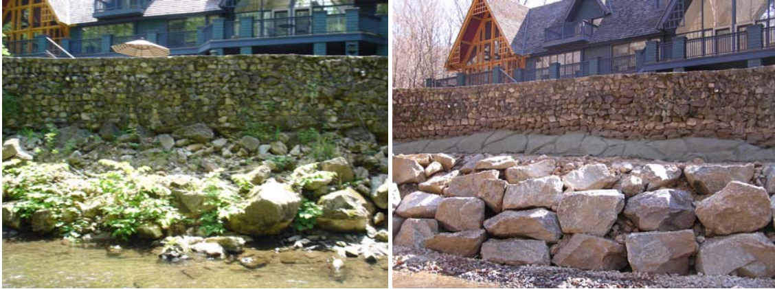
Figure 2: Project #2 Retaining Wall Before and After Restoration
