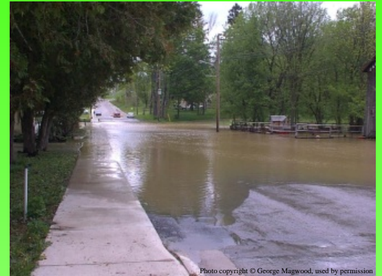
Flooding caused by poor stormwater management
