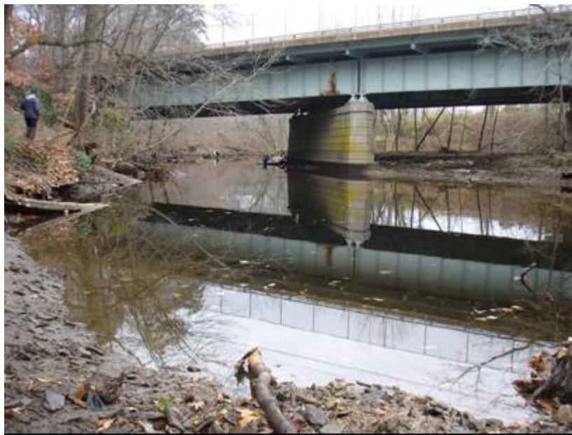
Partially dewatered impoundment, December 2007
