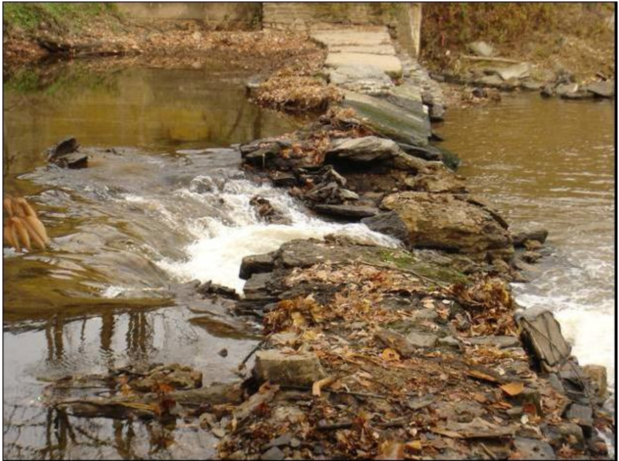
Huntington Pike Dam prior to removal
