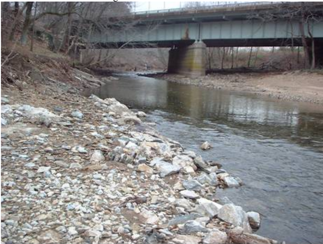
Huntington Pike Dam After Removal
