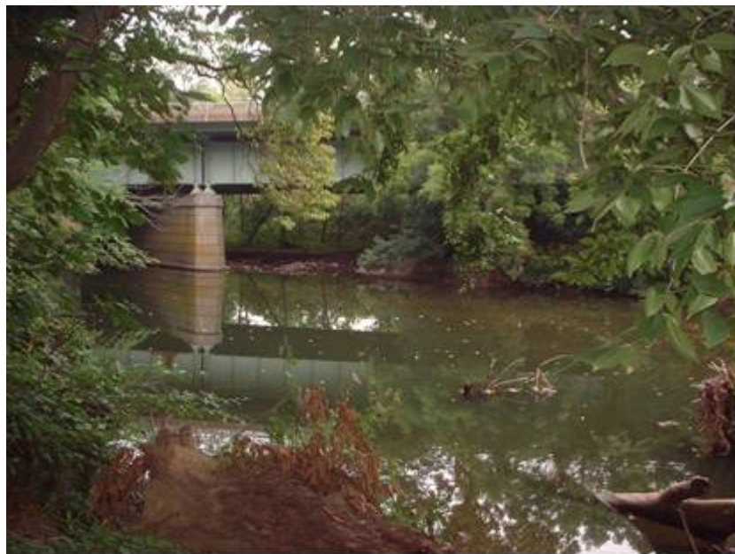
PennDOT Huntingdon Pike Bridge, September 2007
