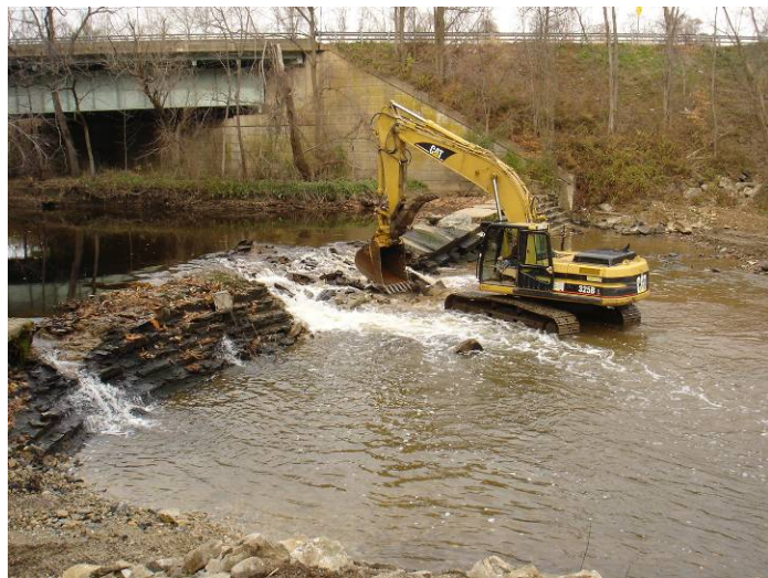
Huntington Pike Dam Removal Construction
