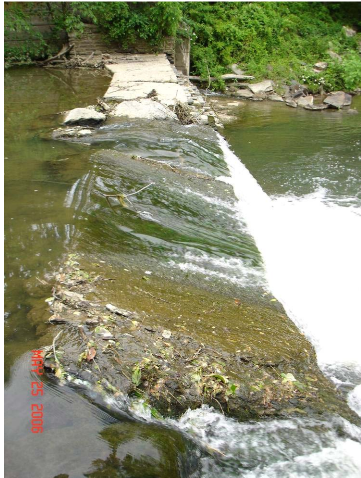
Huntington Pike Dam Prior to Removal
