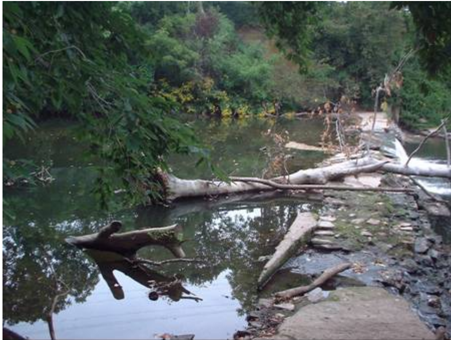
Huntingdon Pike Dam crest, September 2007
