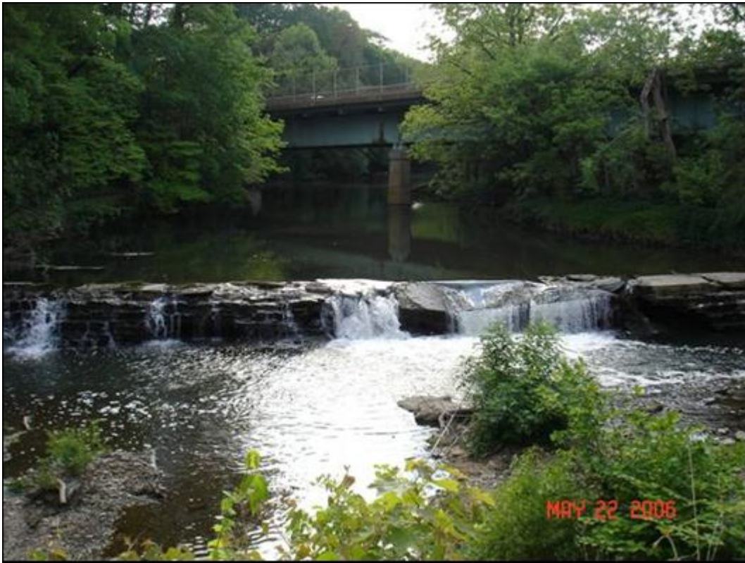
Huntington Pike Dam Before Removal
