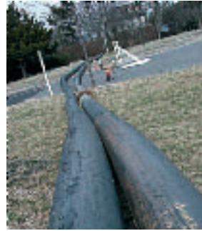
▲ The slurry was pumped 350m to...
