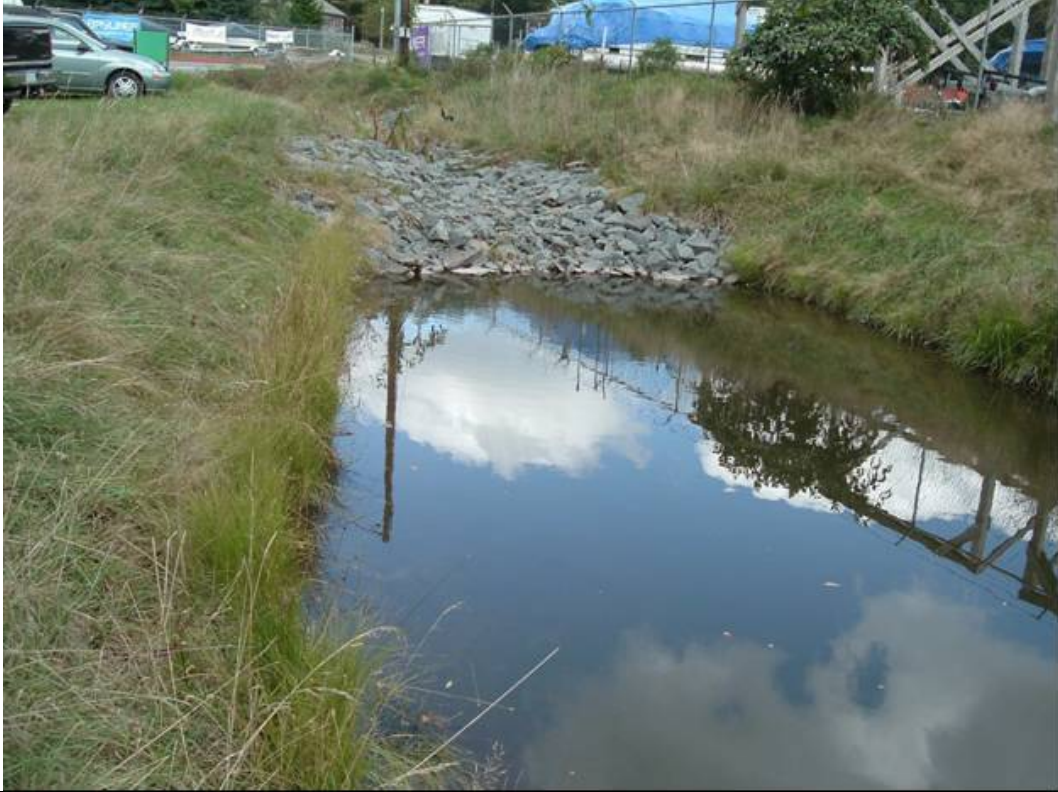
Sediment Forebay at Constructed Wetland Inlet
